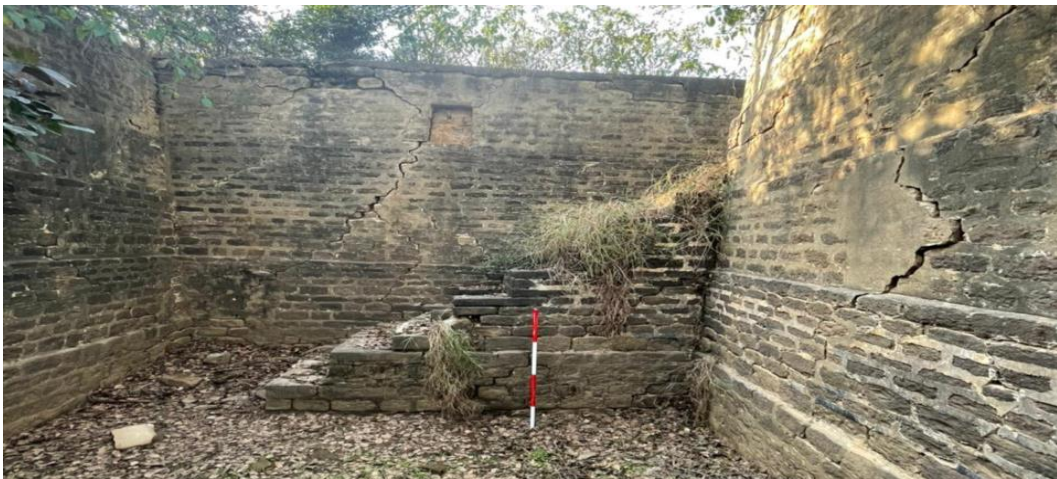
Fig. 6: General view of the Daura Rajgan Tank.
