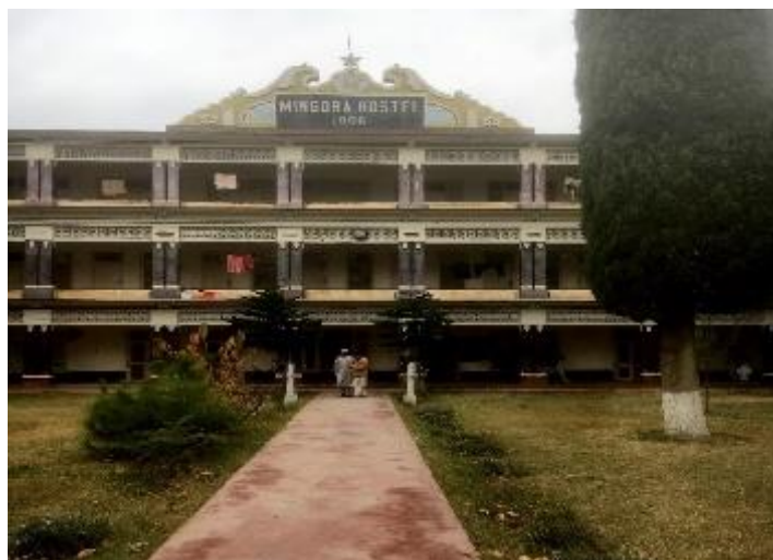
Fig 11: Front façade (Author, 2019)
