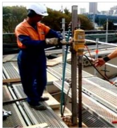
Fig 3: Coring Operations and Bar Post-Tensioning (Branco & Guerreiro, 2011)
