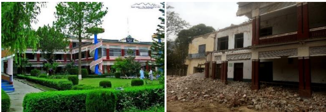
Fig 16: Before and After Demolition of South Block (swat, 2006) (Author, 2019)
