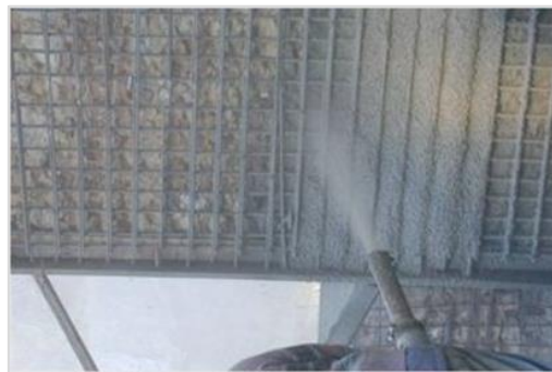
Fig 1: Application of Steel mesh walls & cement grout spraying technique. (Branco & Guerreiro, 2011)
