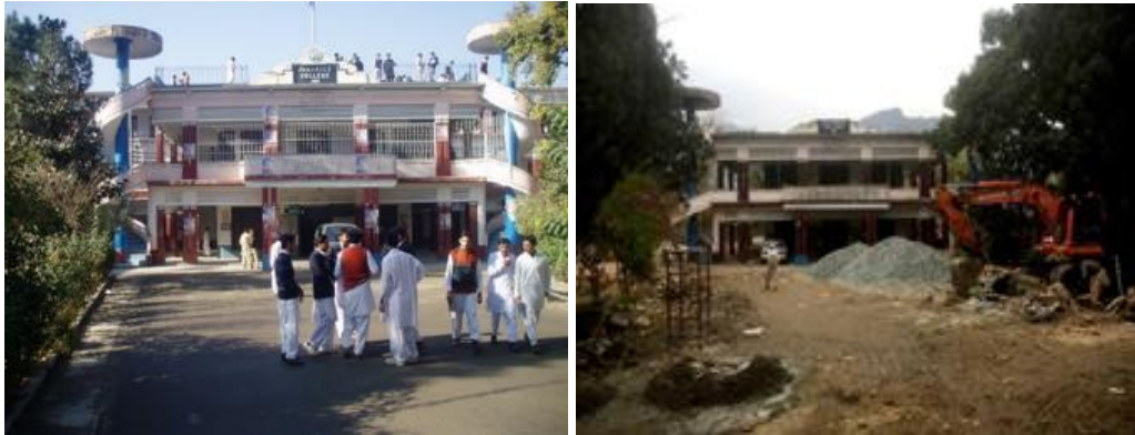
Fig 15: Before and After Demolition for Reconstruction. (swat, 2006) (Author, 2019)
