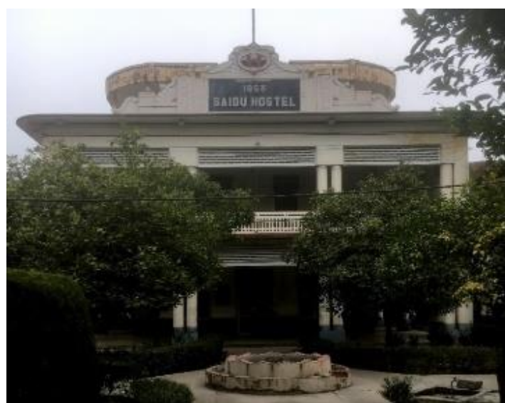
Fig 14: Old building (Author, 2019)
