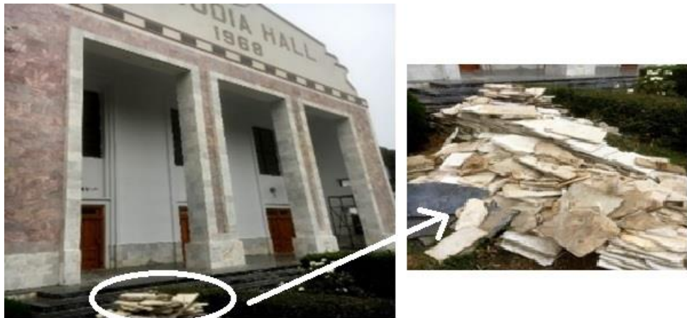
Fig 10: Wadudia hall renovation work in which original tiles were removed (Author, 2019)
