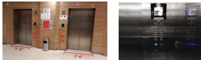
Figure 10 Size and Height of lift, and no Braille Buttons
