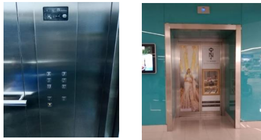
Figure 26 Lifts and Braille Buttons
