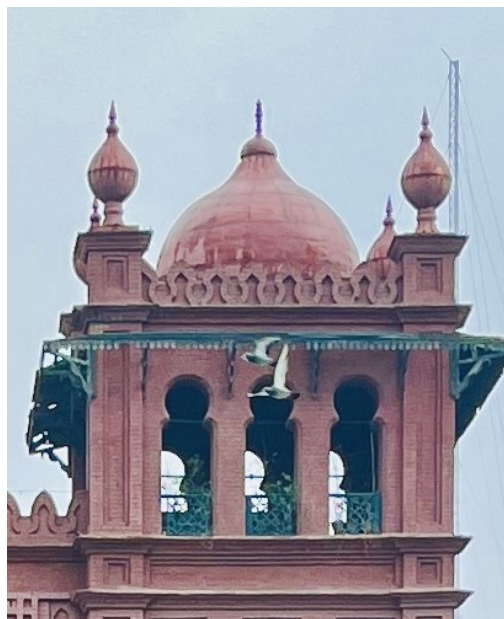
Figure 6: Upper Portion of the Square Tower
