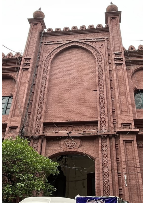
Figure 7: High Arched Frame on the Western Side Elevation
