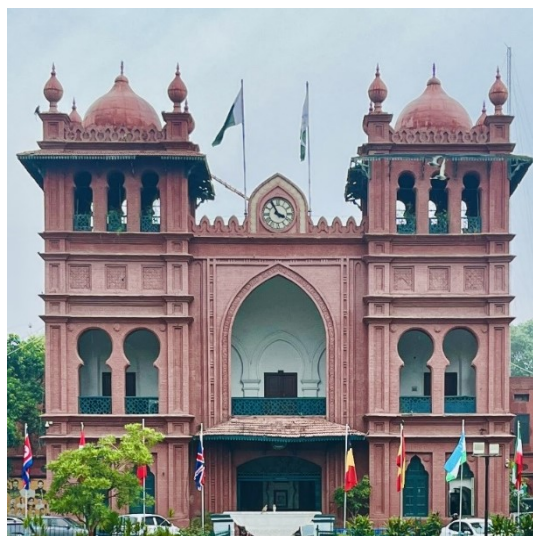
Figure 2: Front Elevation of Town Hall Showing Main Arched Entrance
